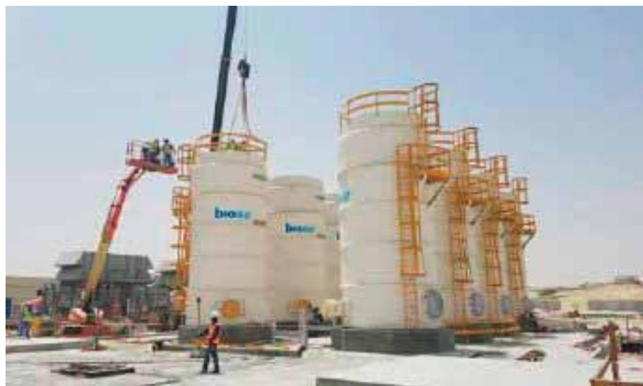
Eight EcoFilter biotrickling filters reactor vessels will treat odors at the STEP project's main pumping station. Photo by BioAir Solutions
